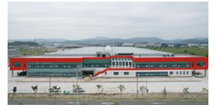
산업설비 (Industrial Facility)
